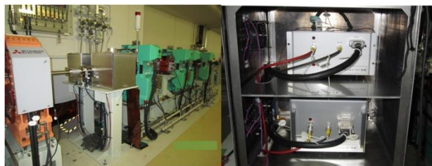
Figure 7: Actual setup of the driving circuits stored in the radiation and noise shield boxes. Two driving circuits are connected to each coil. The one is standby driving circuits.
