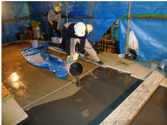
Figure 5: Picture of self-leveling method work.
