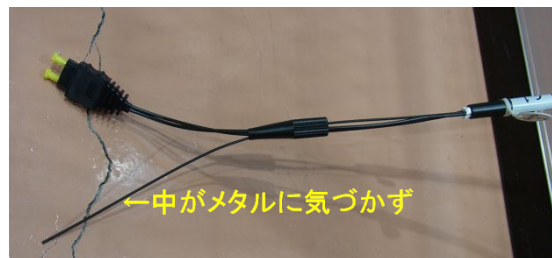
Figure 4: Discharged with this optical fiber cable
