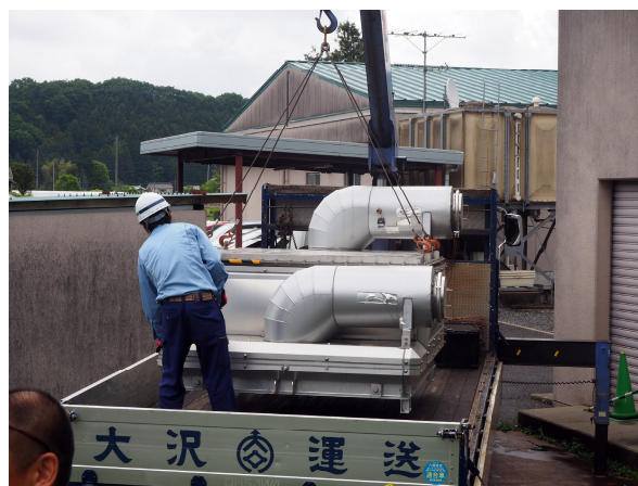
Figure 8: Adsorption thermal storage tank on the truck.
