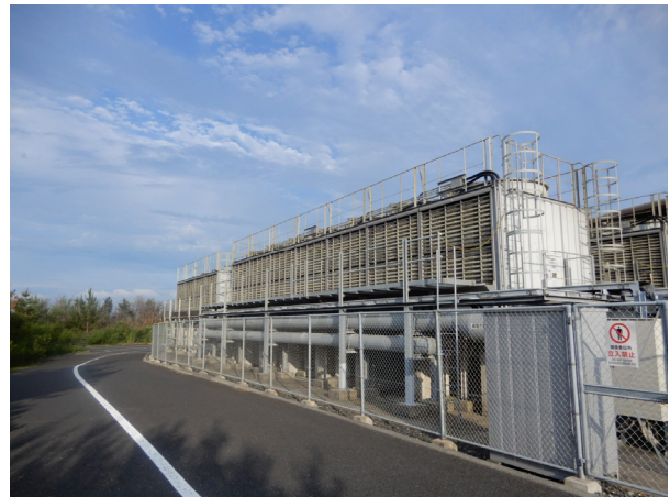
Figure 1: Cooling tower.
