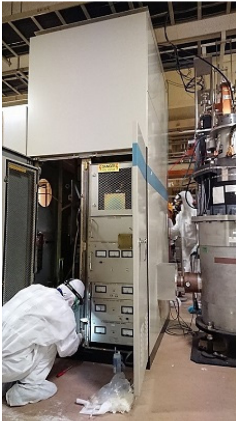
Figure 1: Cleaning work of klystron power supply performed by wearing protective clothing.
