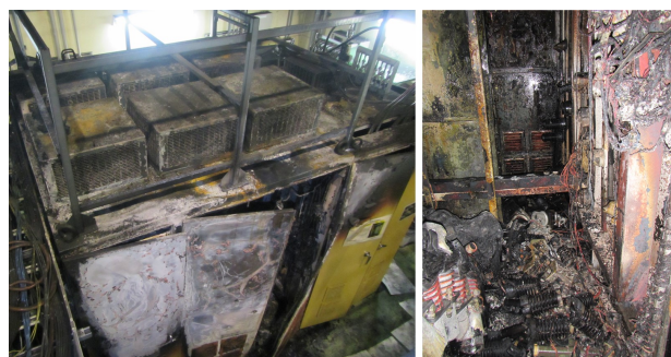
Figure 1: Bird's-eye view (left) and inside (right) of the burnt modulator at Nextef1 (April 2019).
