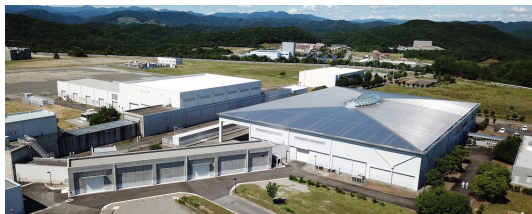
Figure 1: Bird's eye view of the NewSUBARU building.
