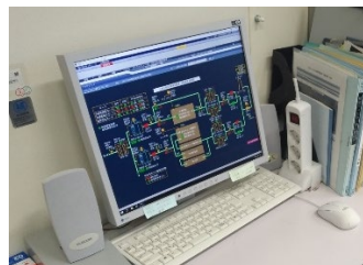
Figure 2: Proprietary workstation in the control room.
